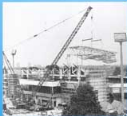
20 Mammoet works on PSV's future
